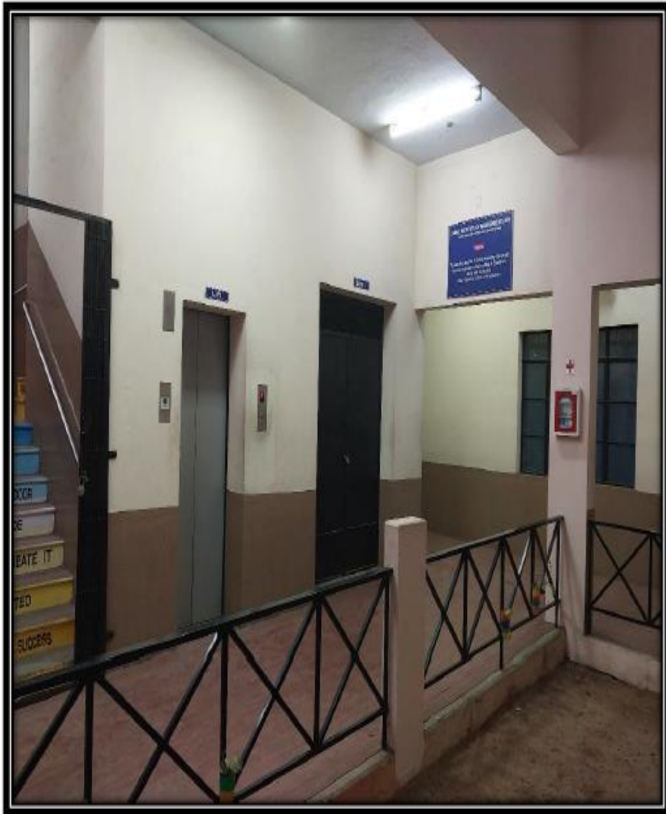
Lift Facility in MBA Block
