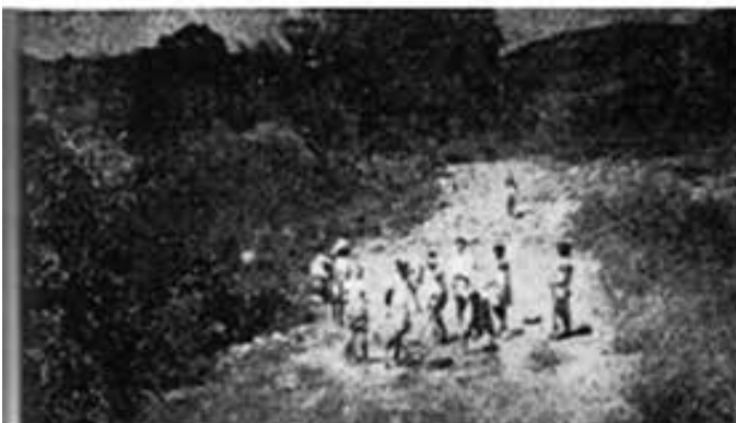
Laying a Road for progress at Pachaimalai
