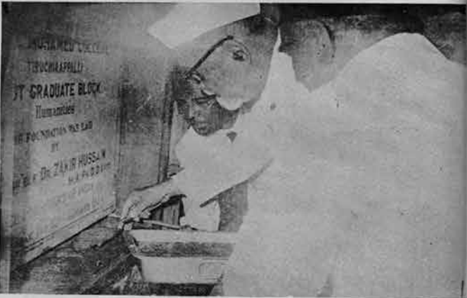
The Vice-President lays the foundation Stone of the Post-Graduate block.
